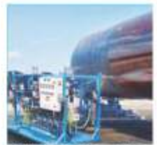
External Automatic Pipe Coating
