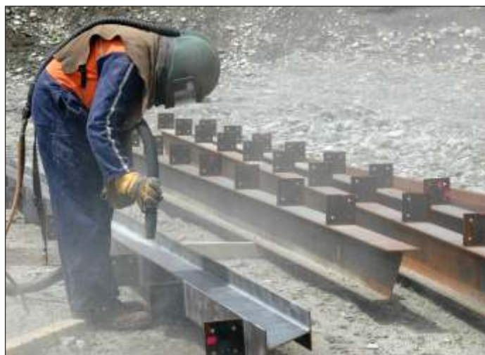
Techniques like sandblasting, power washing, and chemical cleaning ensure optimal adhesion performance.
