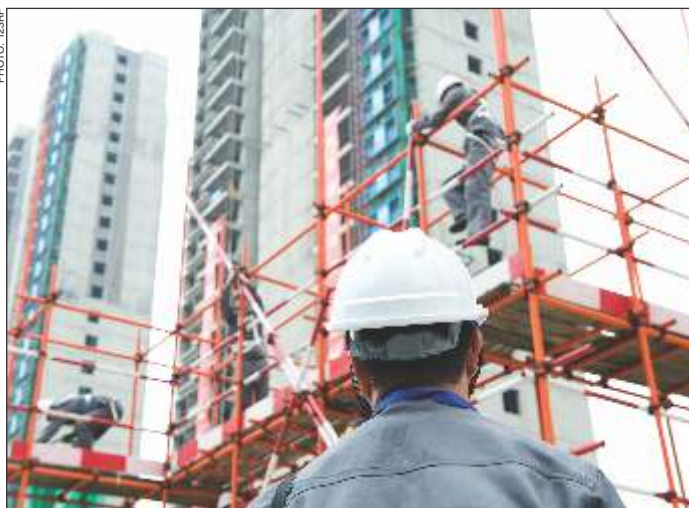
Corrosion can lead to structural failures, posing safety risks in various sectors.
