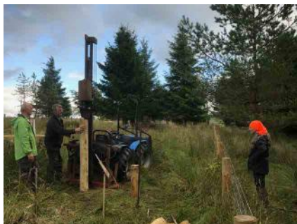
- Driving the piles (Peter Caunt)
