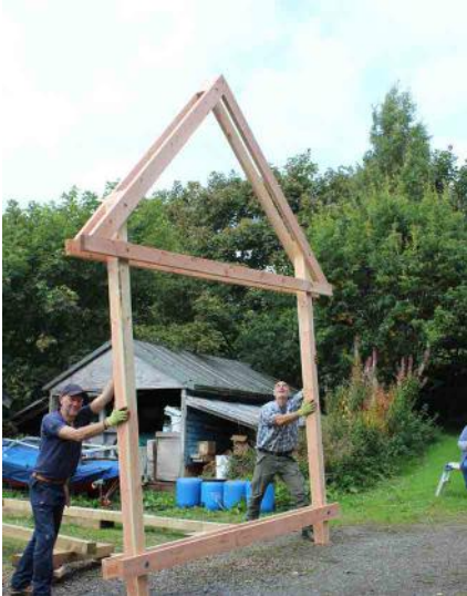
- Frame pre-fabrication at Sunnyside (Peter Caunt)
