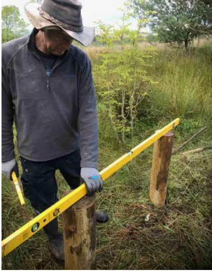
- Levelling the foundations (Peter Caunt)
