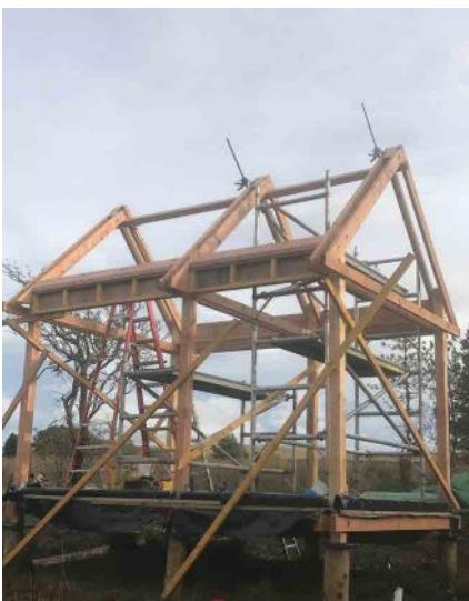
- Frame with temporary bracing (Peter Caunt)
