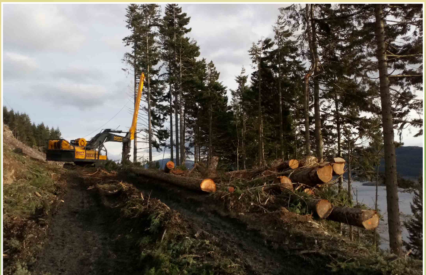
Photo: Cable crane extraction at Primrose Bay
