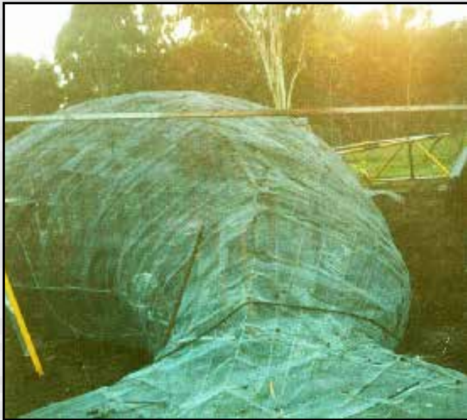
The steel armature ready to receive the first layer of render
