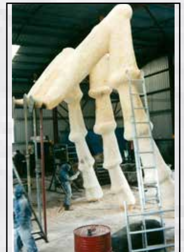
Stage 4 - Building the Legs
