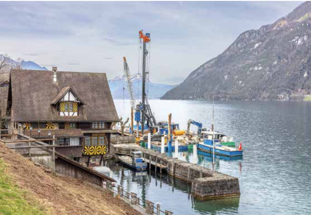
The water construction site in Seelisberg challenges the LB 30 drilling rig with extremely hard rock.
