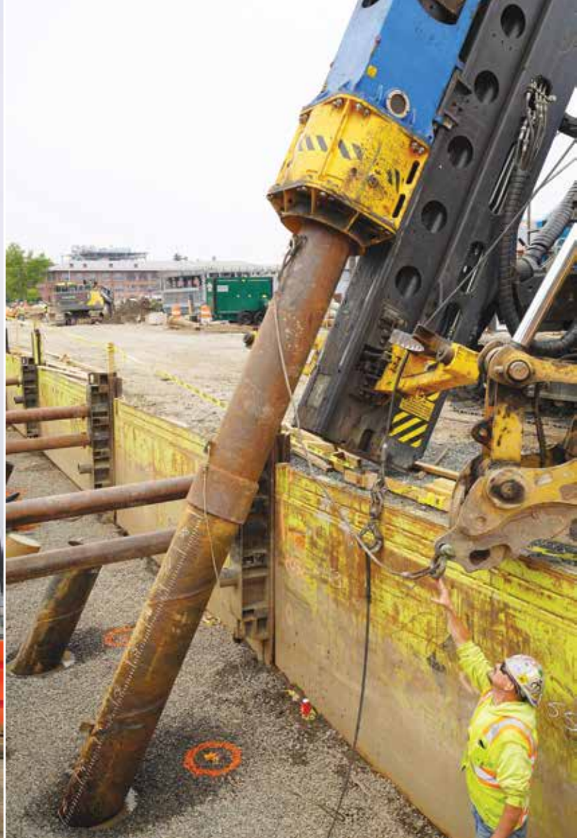
The transition between vibratory and standard pile driving was seamless. Junttan USA equipped the PMx28 with a PTC variable moment hammer and power pack (not pictured) to drive sheet piles, and an HHK5S for pipe piles.
