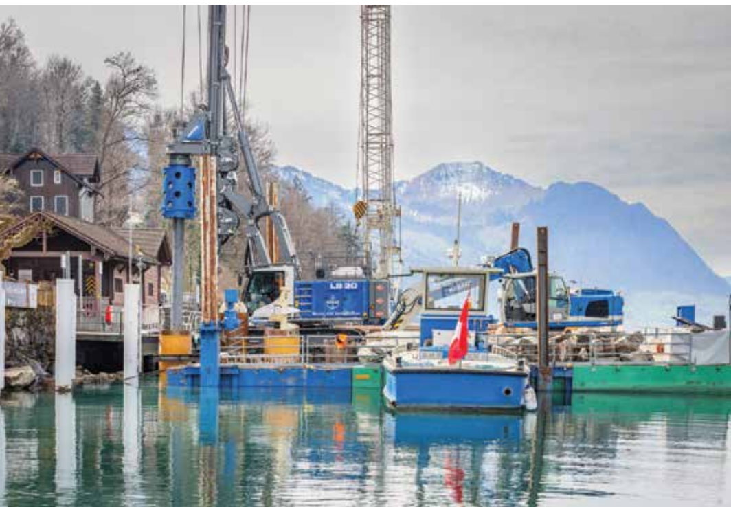
Kibag is using the LB 30 to install new mooring piles for the Lake Lucerne Navigation Company.
