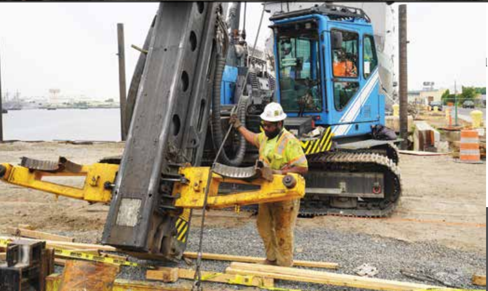
Junttan USA conducted a stability analysis to ensure that the PMx28 would stay upright while supporting an 8,000-pound pile and 23,500-pound hammer while holding an extreme 2V:1H batter.
