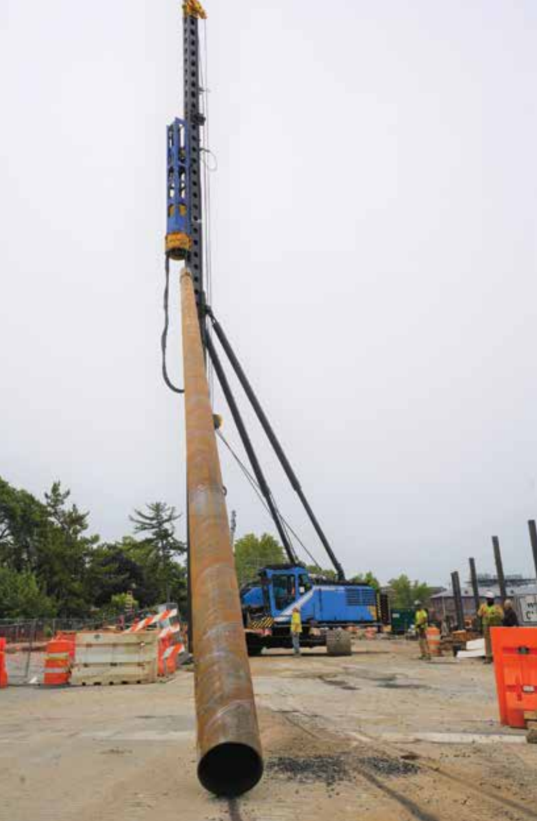
The PMx28's ability to hoist and drive piles without falsework was the main factor for JJA choosing the Junttan rig over its traditional use of a crane-mounted hammer.
