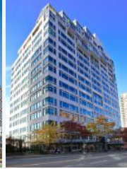
Market Place Tower CBRE
