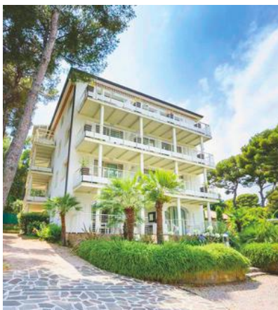
ROQUEBRUNE CAP MARTIN APARTMENT BUILDING
