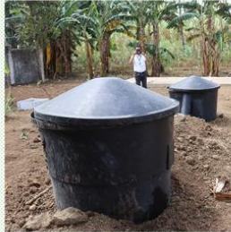
Biogas Digester
