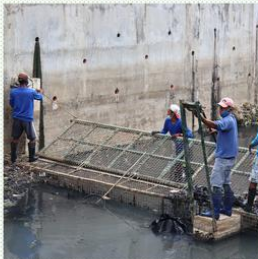
Fabrication and Installation of Trash-trap, Trash-net, and Composting Facility
