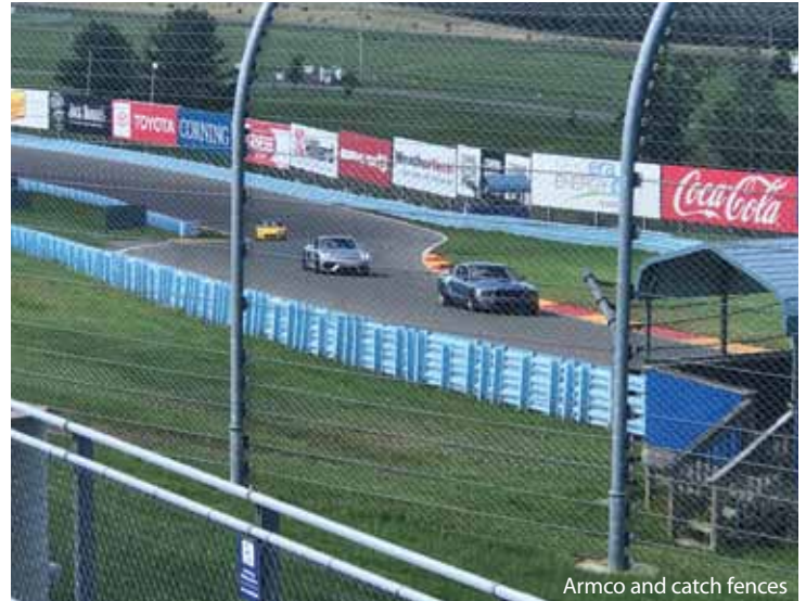
Armco and catch fences
