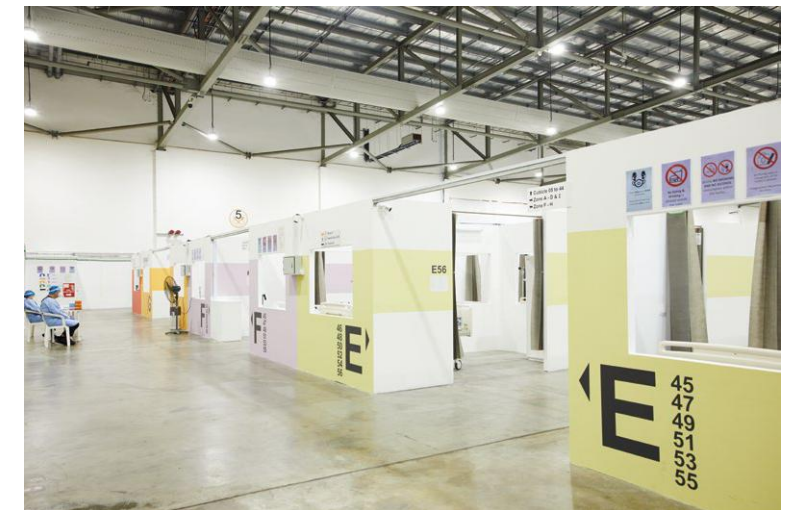
CCFs were organised by zones, and the blueprint drawn up by the public sector was later used by the private sector to build more facilities.
