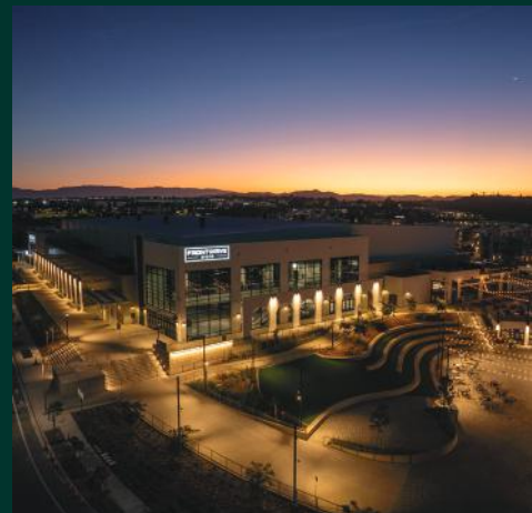
FRONTWAVE ARENA Pascal Steel Coporation Oceanside, CA
