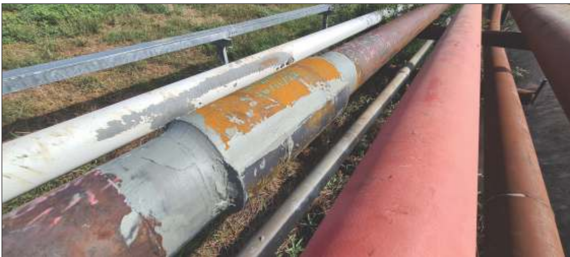
The completed application restored strength to the pipeline wall.
