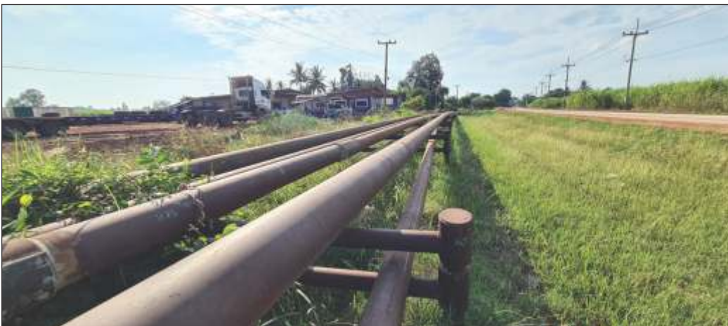
Belzona repaired a pipeline made out of 12 metre pipe lengths in the petrochemical industry using cold bonding.
