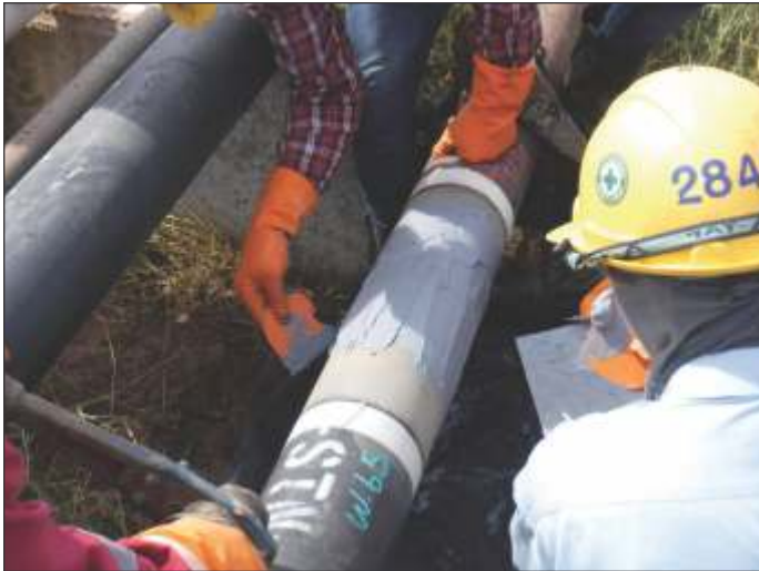
Belzona 1111 (Super Metal) was applied as a bonding agent.
