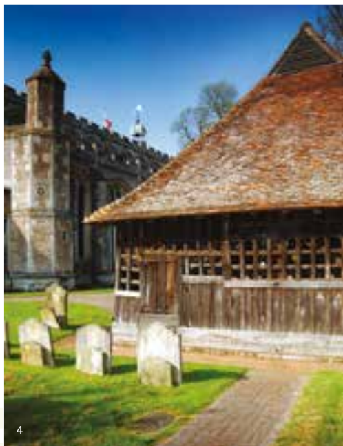
1. Willy Lott's House 2. Sign in Dedham 3. Bridge Cottage and Flatford Bridge, Flatford 4. Bell Cage, East Bergholt Church 5. Sir Alfred Munnings Art Museum 6. Rowing boats at Dedham
