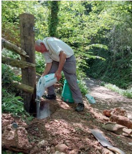
Post-Fast is poured into the hole.
