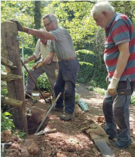
An absolute essential – posts must be upright or they are no use at all!
