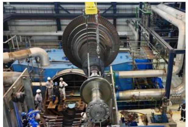
Lifting of Steam Turbine Rotor During Major Inspection
