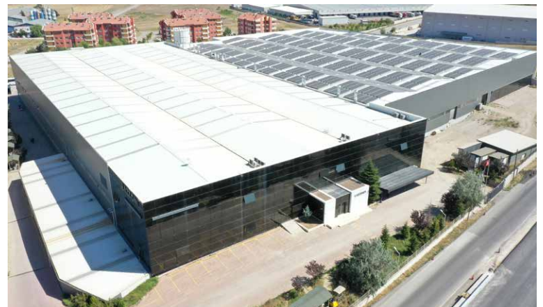
Headquarters in Ankara, Turkey. First modern manufacturing facility. 2002
