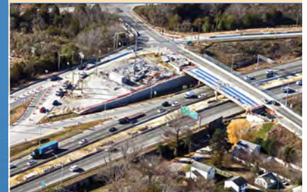
MALLORY STREET BRIDGE
