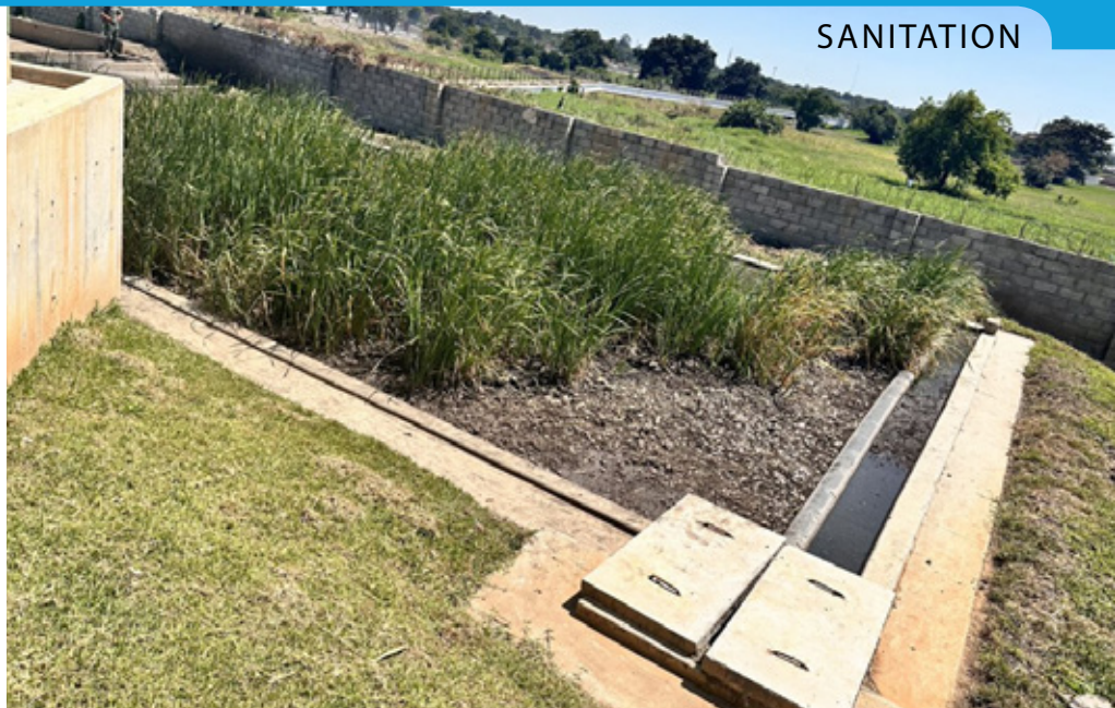
Wetlands used to treat liquid fraction from faecal sludge treatment plant, Zambia
