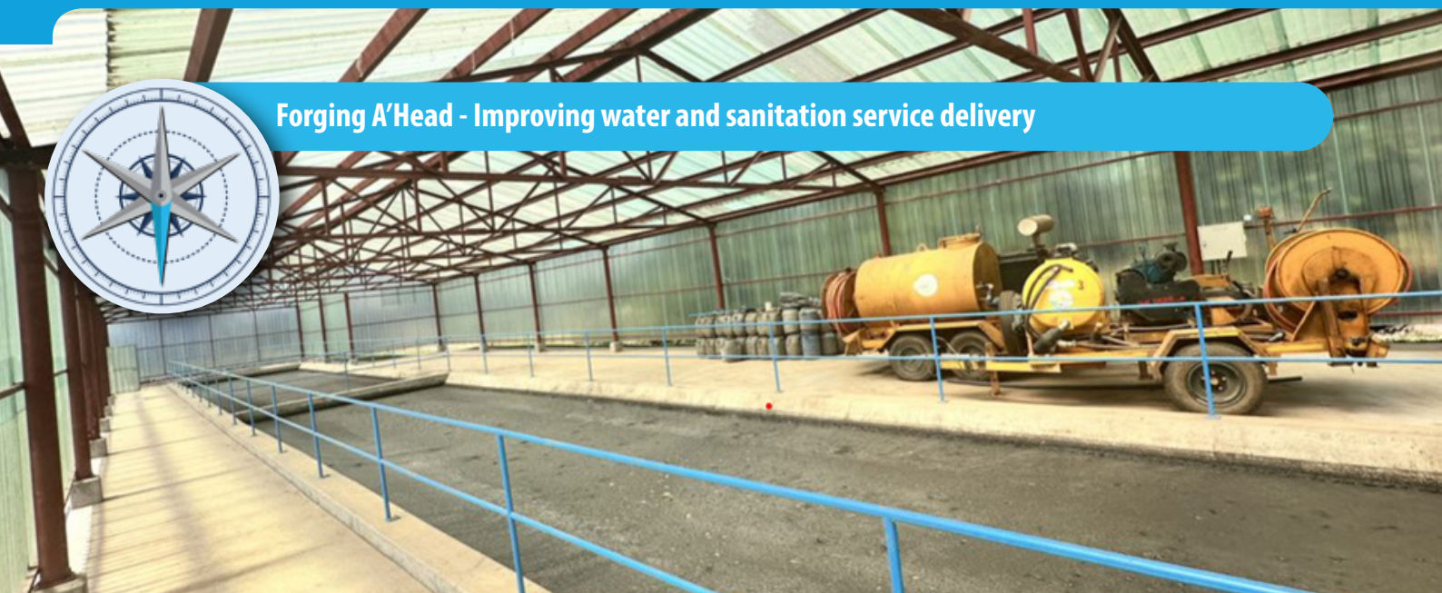
Faecal sludge treatment plant, Zambia
