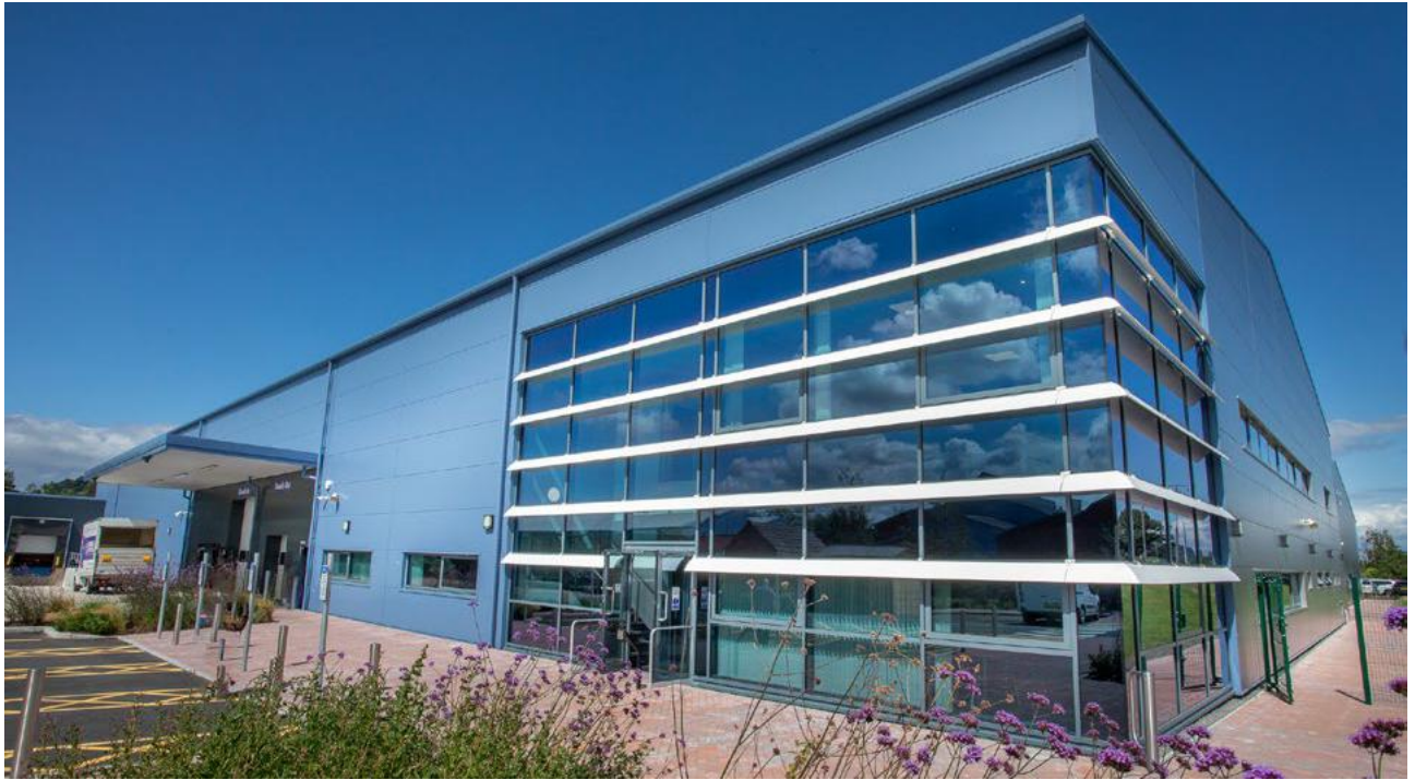
Invertek Drives, Welshpool Production & Warehouse Facility, BREEAM Excellent
