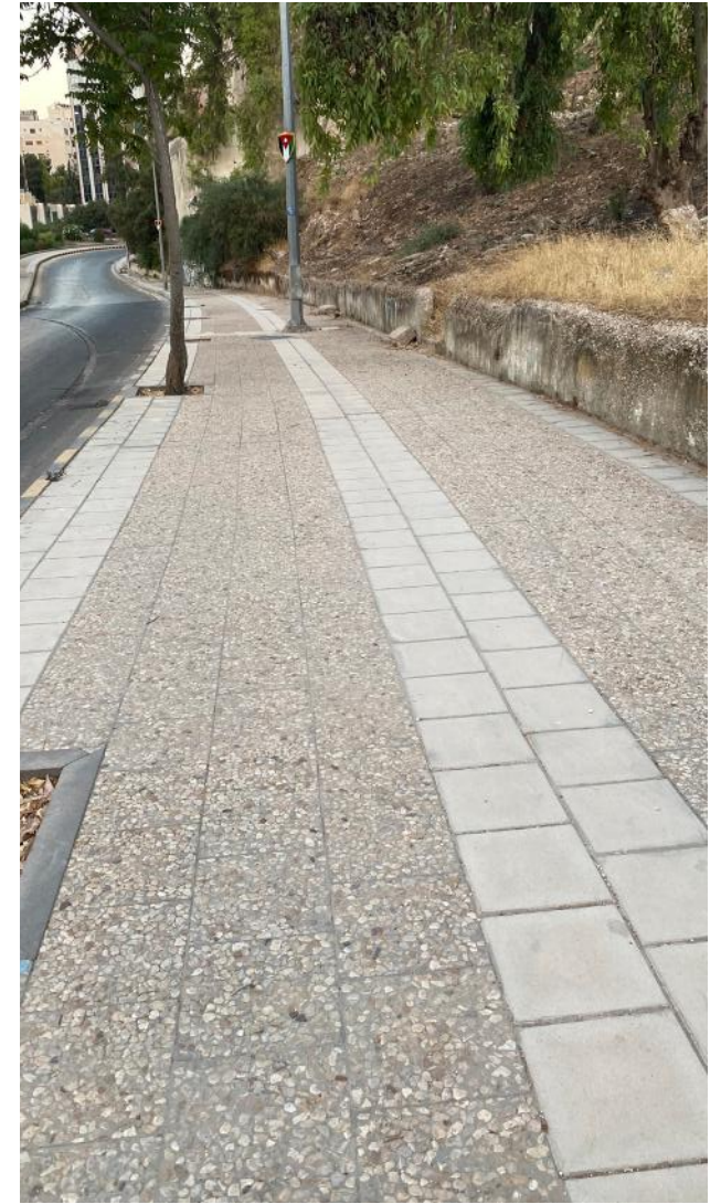
Exposed aggregate concrete tiles and plain concrete tiles on a side walk along Arar Street in Amman.
