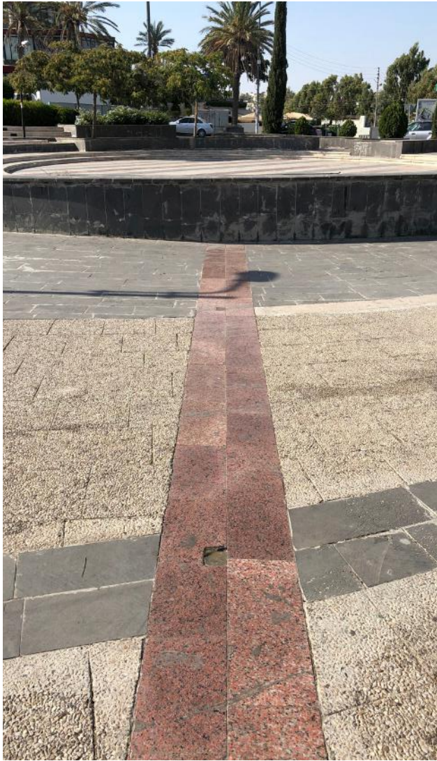
Exposed aggregate concrete tiles, basalt stone, and granite paving materials. Combining stone elements with concrete tiles adds visual interest and is more economical than exclusively using stone paving. The photo is of the paving in 'Abdun Circle in Amman.
