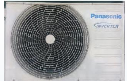
R410A split air-conditioning unit converted to RS-53 (R470A) & operating satisfactorily without any problems
