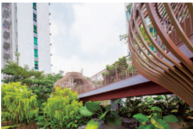
Linking the tree houses is the Tree Top Walk, the ideal place for a romantic stroll in the evening. With ethereal lights illuminating the path, the tree houses come to life at night as the soft glow through the arches creates a mystical tapestry of silhouettes.
