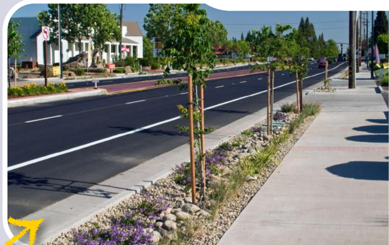
The above image depicts what a walkable streetscape should look like, including wide enough sidewalks with a buffer from the roadway and landscaping including street trees for shade and aesthetics.
