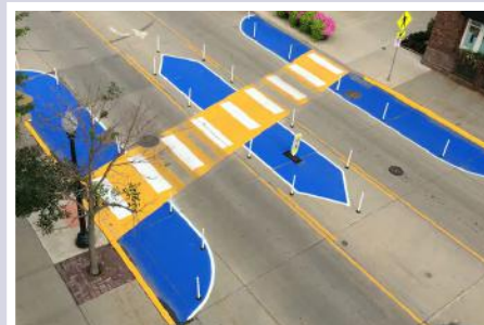
Safety measures at road intersection crossings can include active measures such as pedestrian signals (left) and passive measures like curb extensions (above)
