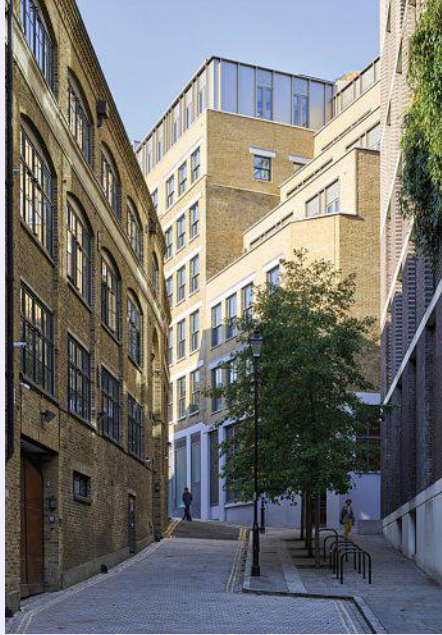
Above Rear elevation looking up from Crawford Passage. To avoid planning concerns, new external terraces sit within the former building line of what was a more recent, curved mansard.
