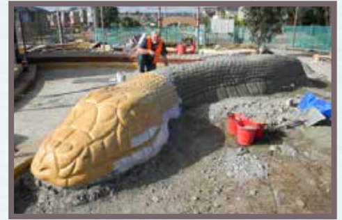
First Coat of Paint being applied - Image 3
