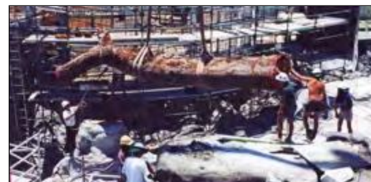
Artificial Rock steel Armature
