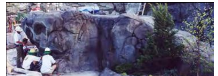
Artificial Rock work in progress
