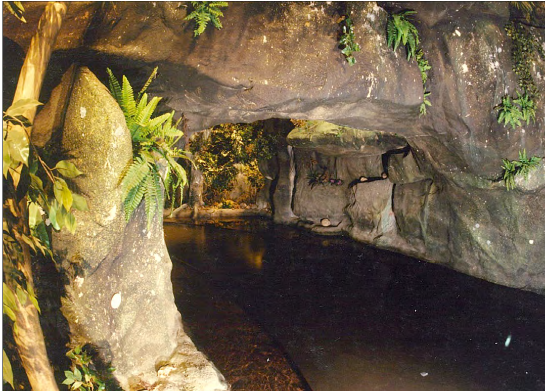
Artificial Rock & Plants - during construction of boat ride
