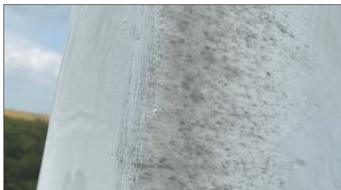
Successful application of Belzona polymeric systems.
