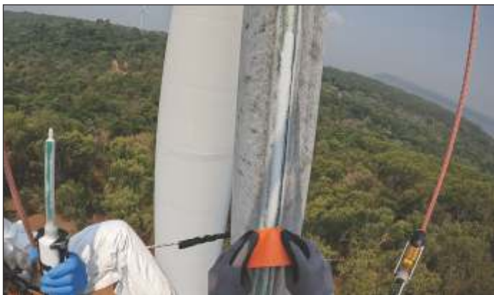
Application of repair paste, Belzona 5711.
