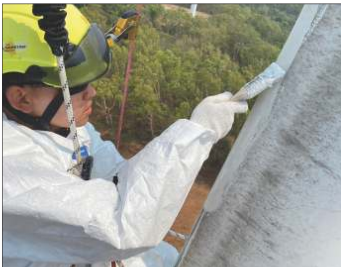
Application of high-performance coating, Belzona 5721.
