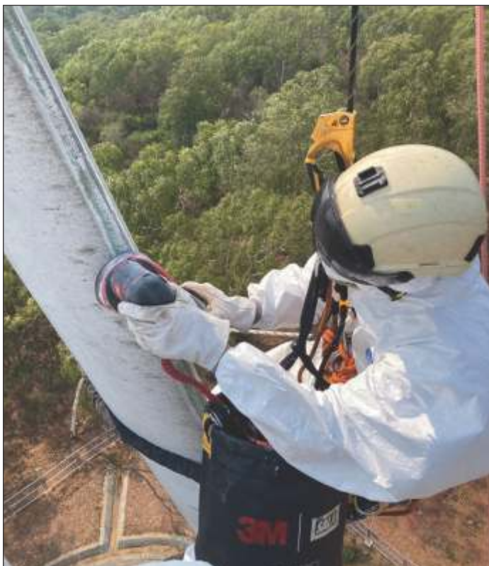
Surface preparation using an orbital sander.
