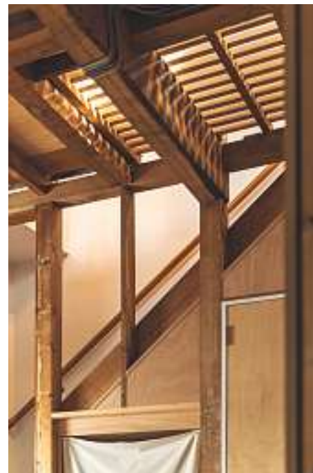
Above: At Haruka Nogami's home, new structural insertions, such as light-permitting slats, were in cypress.
