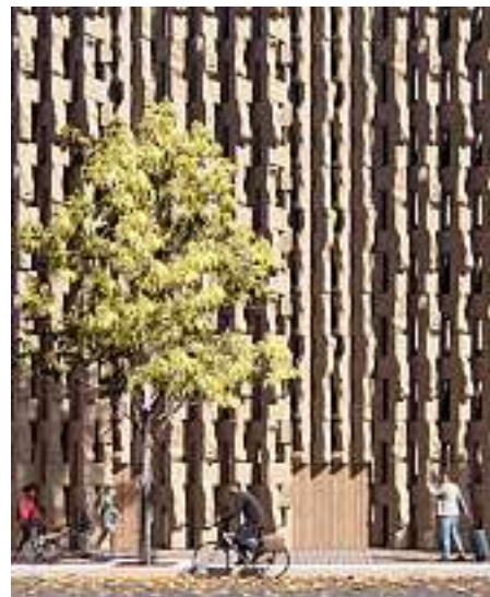
Above: AI can be used to scan unpredictable material such as reclaimed stone, and design around it – as on this Oxford Brookes student project.
