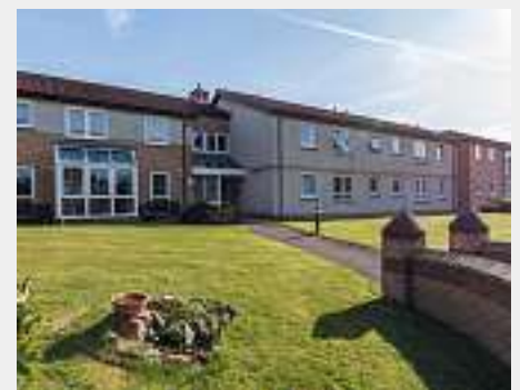
Above: Sidey replacement project.
