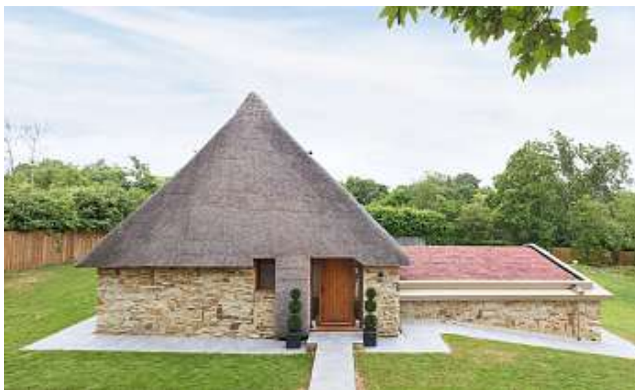
Above: Thatching in progress at Thatch House, Cambridgeshire.
