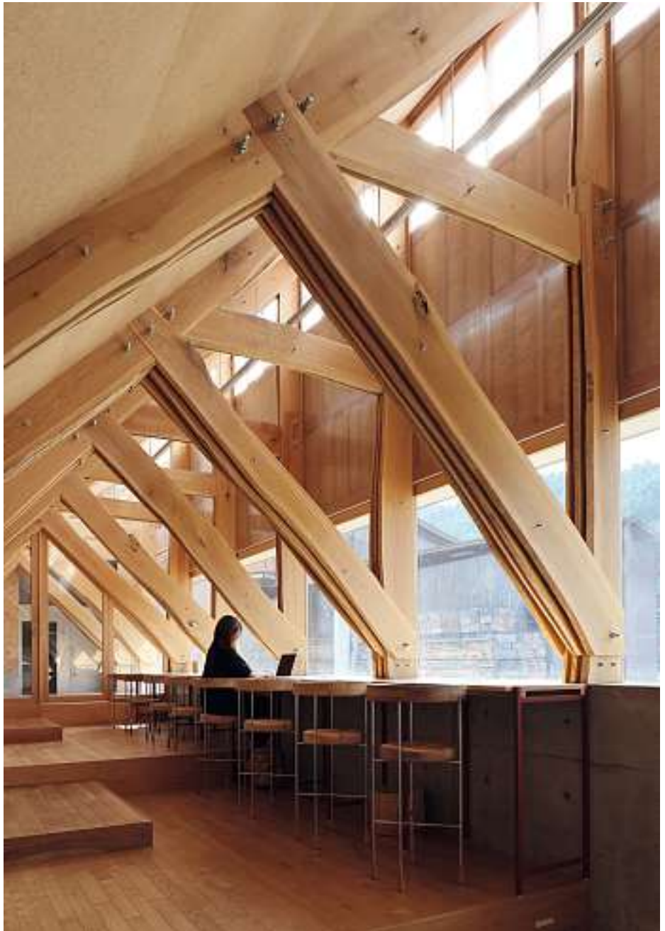
Below: At Morinaha, raw sections of timber are cut to the same thickness, giving a unique profile to each mechanically cut piece.
