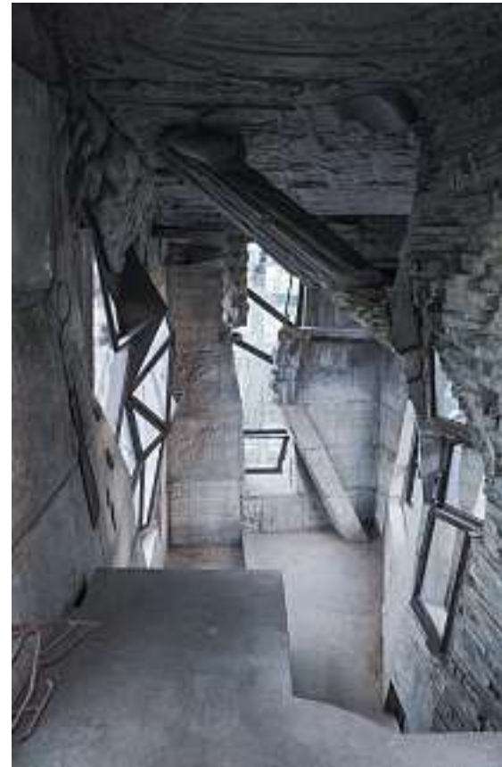
Below: Looking down from the 4th floor to the 3.5th floor. Amateur ‘crafting’ of concrete has given a Gaudi-esque feel to Oka’s home.
