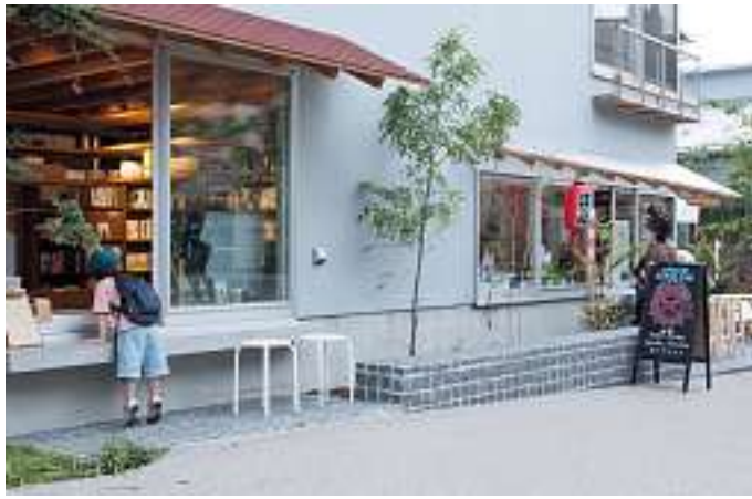
Left: Tsubame Architects used prefabricated house systems for its Bonus Track shops and flats, then added frame elements to let users tweak details.
