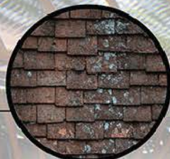
Terra cotta roof
