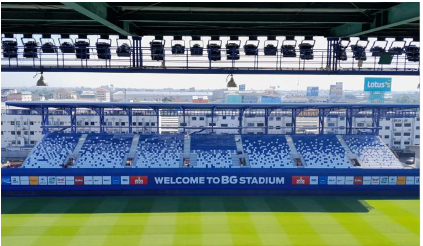
International Project 2024 : 5000 seats grandstand for stadium in Bangkok, Thailand
