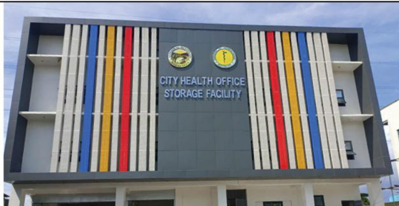
City Health Office (CHO) - Storage Facility
