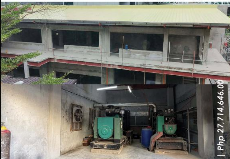
MRF & Toxic Waste Storage at OsMun
