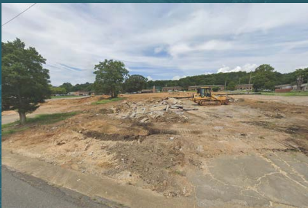
Existing Site Condition
