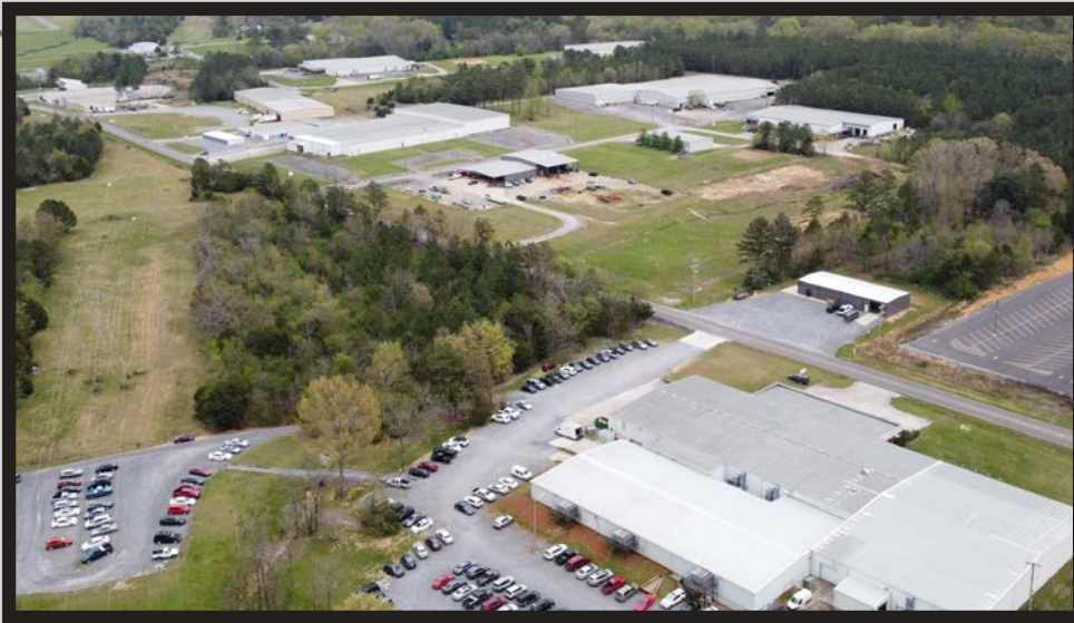
Industrial developments on Airport Rd
