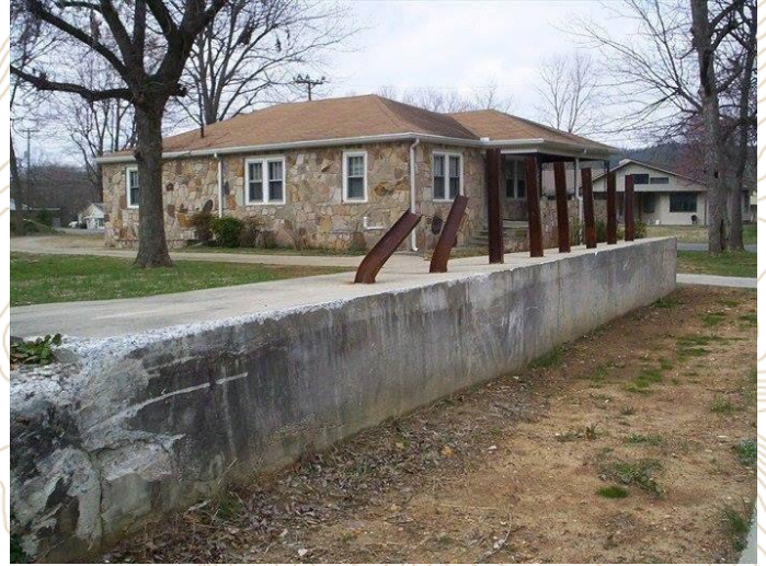
Dangerous concrete barrier for stopping runaway trucks
