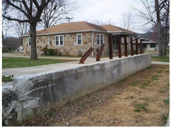
Dangerous concrete barrier for stopping runaway trucks
