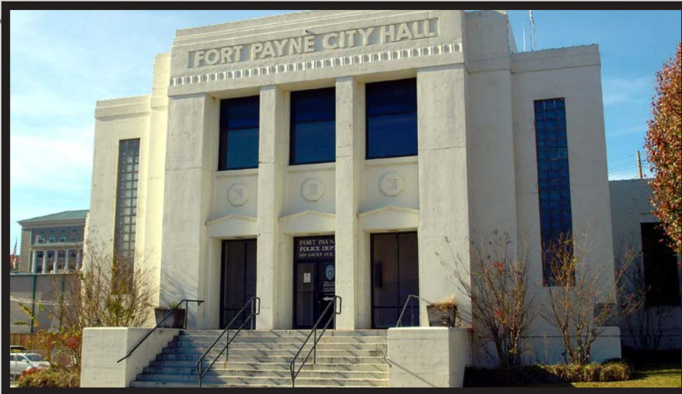
Fort Payne's historic City Hall on Gault Ave
