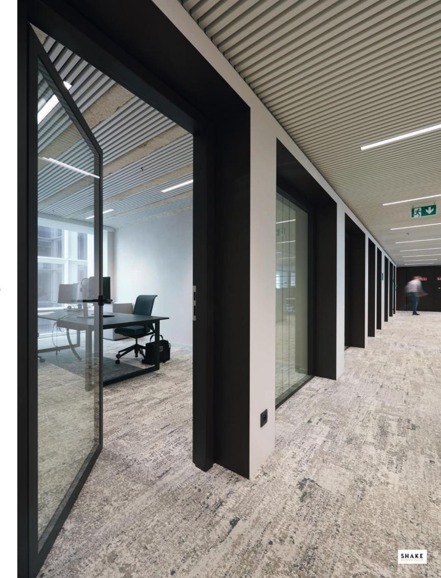
The positioning of the JB PURE 100 glass partitions is unique. Strategically set approximately 30 centimetres back from the plasterboard partitions, this intentional design choice allowed us to craft recessed niches seamlessly integrated into the architecture.
