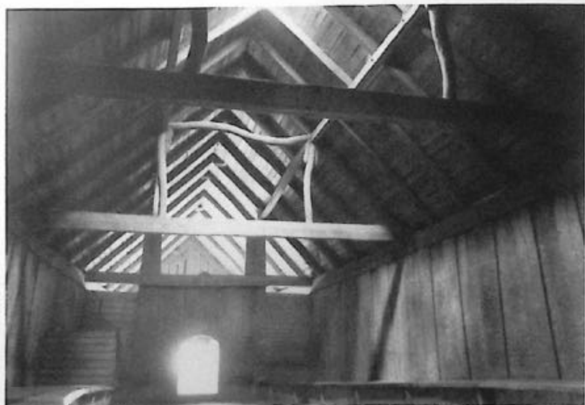
Interior reconstruction at Trelleborg, built following the pattern of the original foundation post holes
