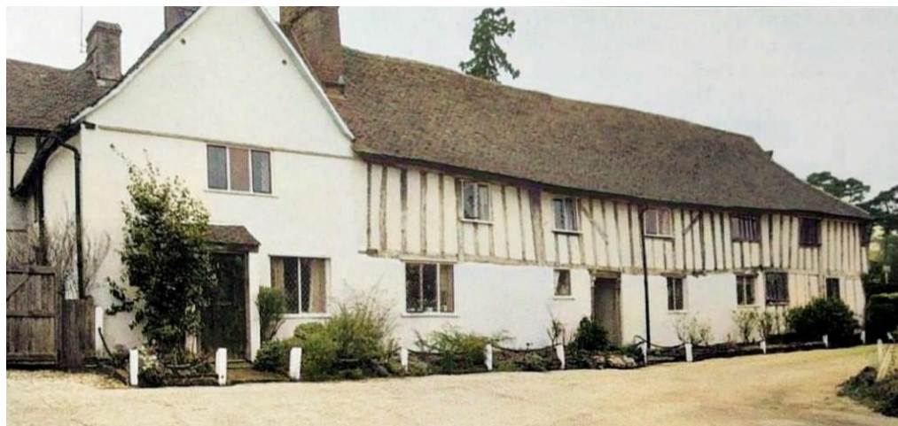
East Front after restoration.
