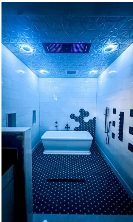
This project was completed for Platow Home and Tile and included a fully waterproof system and custom foam pan.
