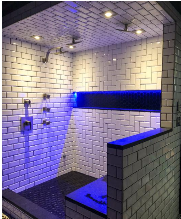
Timeless Construction was Struzik's very first company. He installed this custom steam shower with LED-lit infinity niches.
