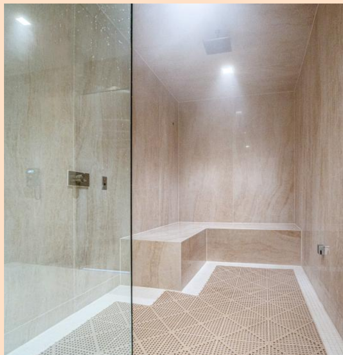
Steam room interior—waterproofed with KERDI-DS.
