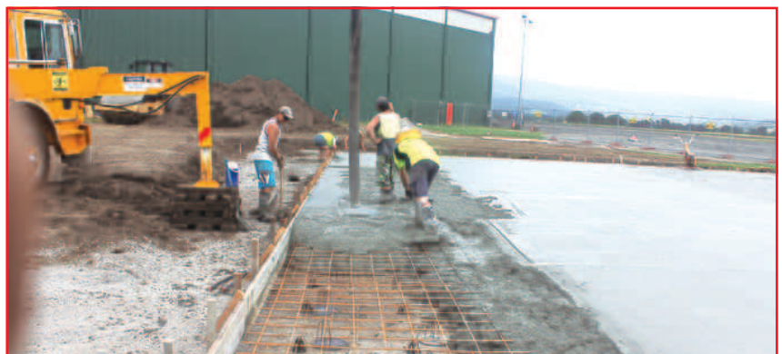
Concrete pouring of the 20 x 20mt slab commences.
