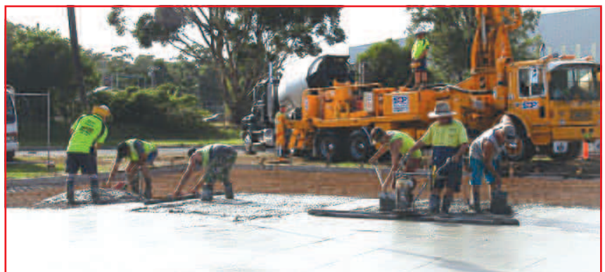
Smoothing out and finishing process.
