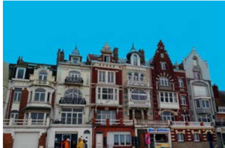
Malo-les-Bains - architecture malouine
