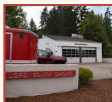
South Shore Fire Station 1880 South Shore Boulevard
