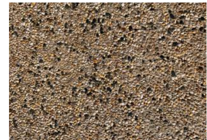
F) Driveway & Paths Exposed Aggregate with 300mm Paths
