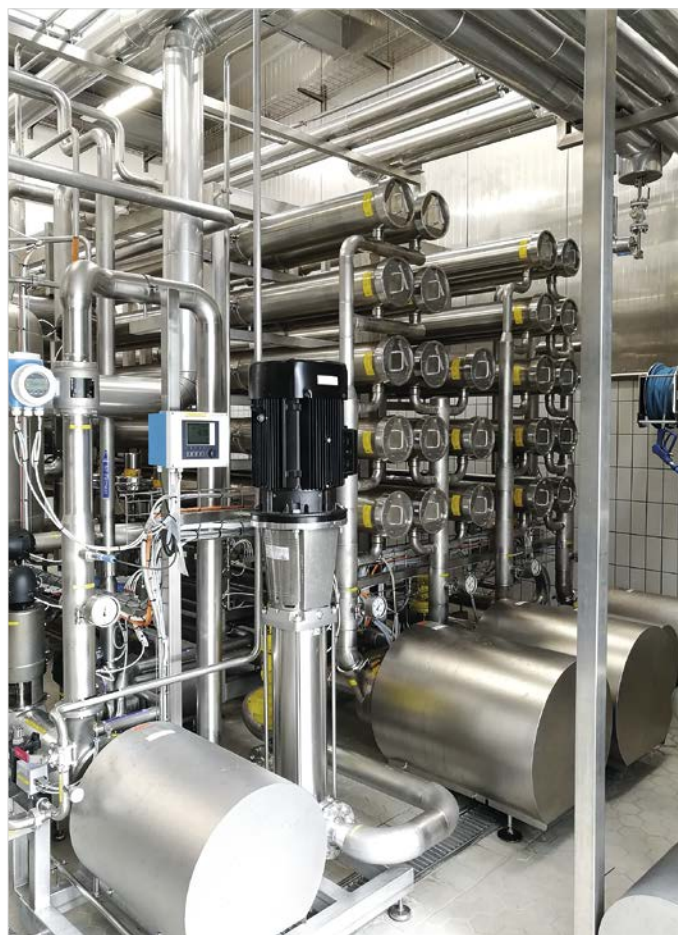
Nanofiltration plant for mozzarella whey (ALPMA) at the customer's site
