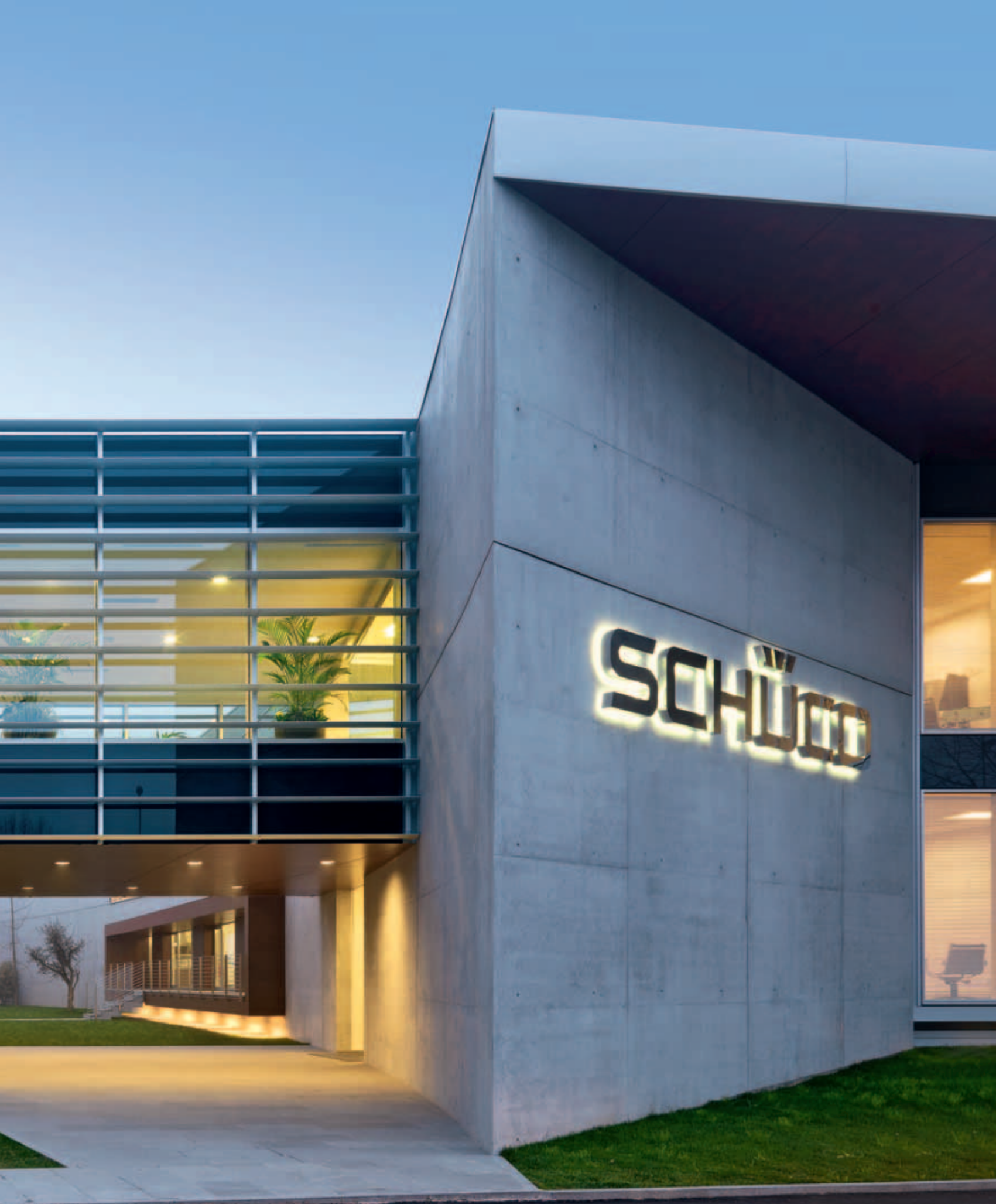
Green Building - Schüco Italia srl Headquarter, Padova, Italy
