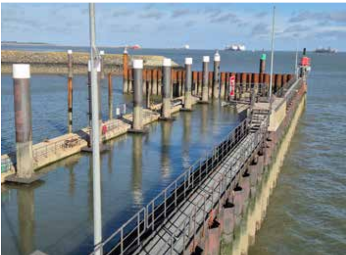
Figure 23: Tugboat harbour of the Jade-Weser Port Wilhelmshaven
