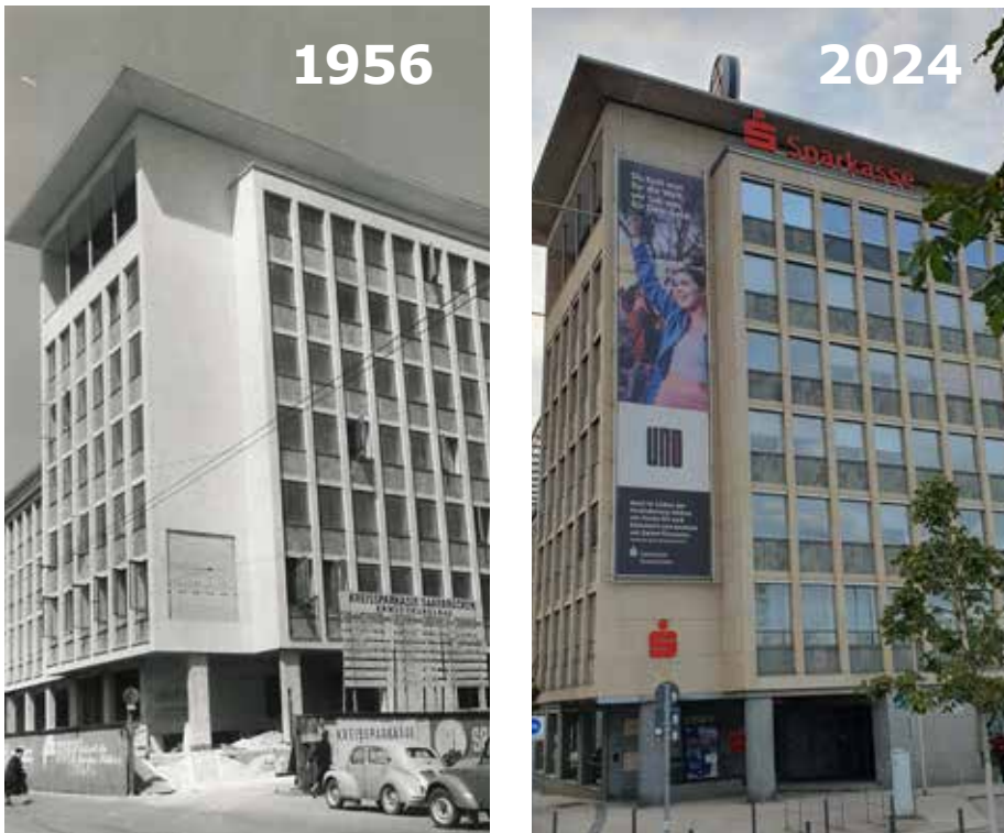
Figure 22: Saarbrücken District Savings Bank, built with supersulphated cement "Halit" from the former "Halberger Hütte"
