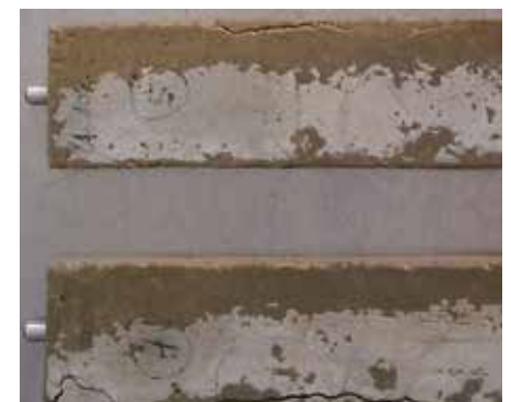
Figure 7: Cracked mortar test specimens with GBS 234 at a GBS/CL ratio of 50/50 after 3,650 days at 20°C
