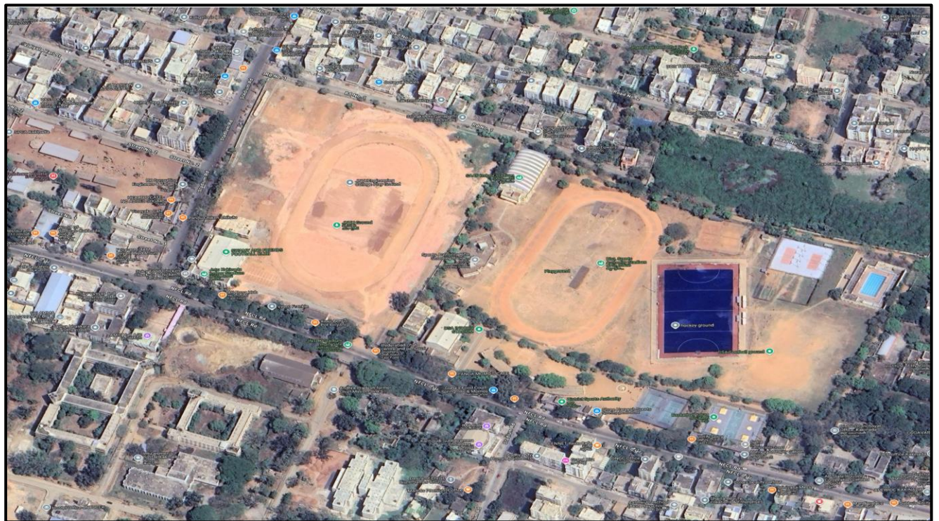
Fig 7: Ortho Rectified Image of JNTU Ground, Kakinada
