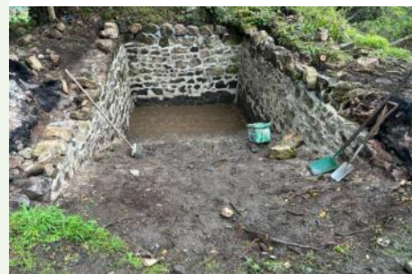
Lime mortar is used to rebuild the side walls.
