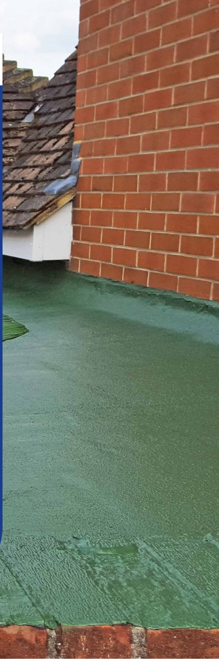
Roof: Super-Flex Green
