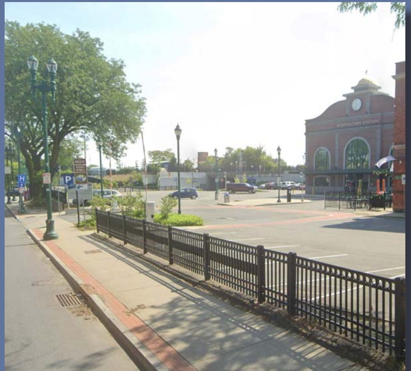
Median dividing the parking lot at the Rensselaer Amtrak Station. Decorative fencing supplements the division of space.
