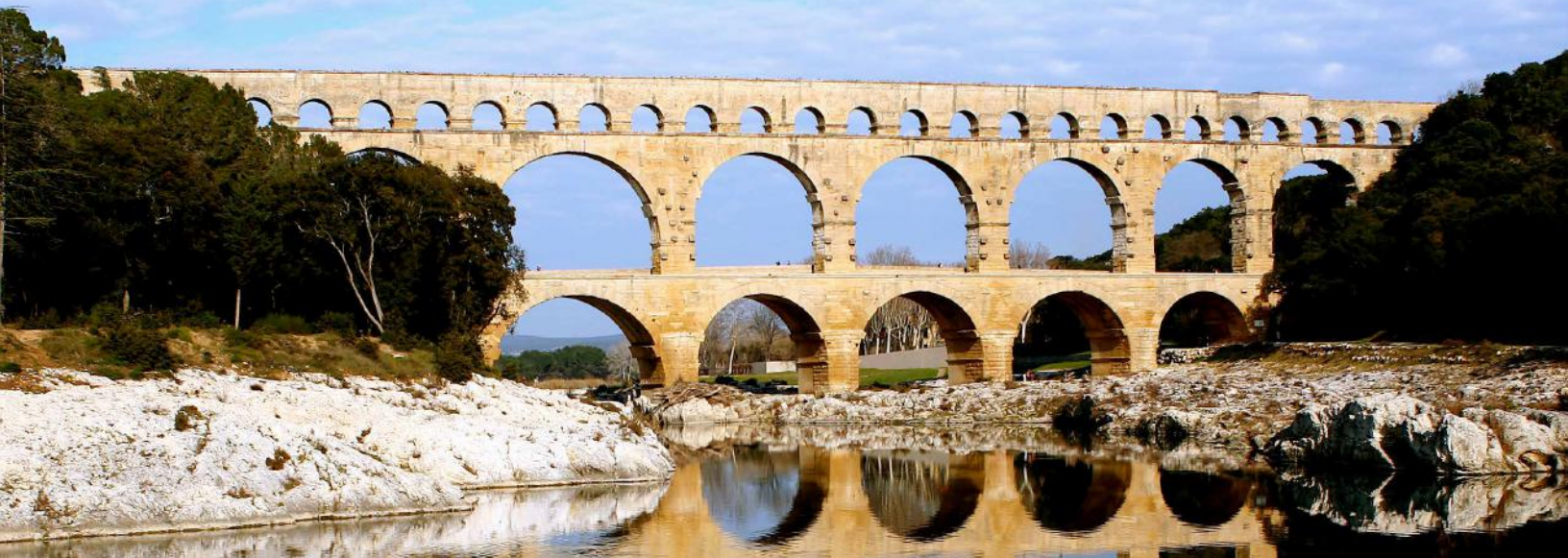
The Pont du Gard in southern France is the highest Roman aqueduct bridge in the world.
