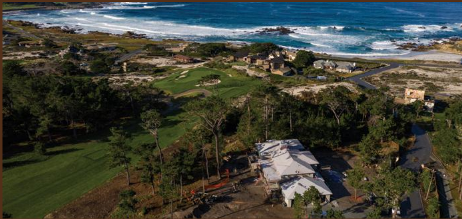
New Construction on the 6th Hole at Spyglass Hill Golf Course
