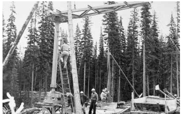
Apex Poma Lift bullwhell under construction during the summer of 1961.
