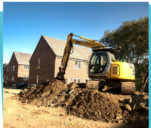
Constructing new homes
